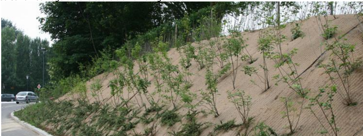
Figure 25 Merlon planté
